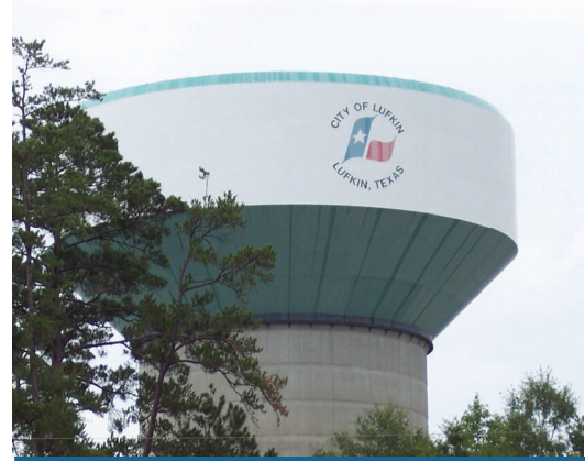
Water Storage Tank on Whitehouse Drive
