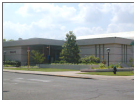
ILLUSTRATION 5-2 The Lufkin Police Department Facility
